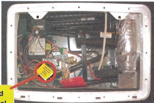
**Retrofitted with thermal sensor # R-010**
